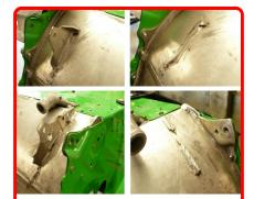
**Step 2:** Remove both existing heat exchanger tabs (left & right). Use of a Sawzall, Dremel c/w cutting disc or similar tool required. **WARNING:** Use extreme caution to not cut into the exchanger. Cut above welds and grind where necessary for clearance.
